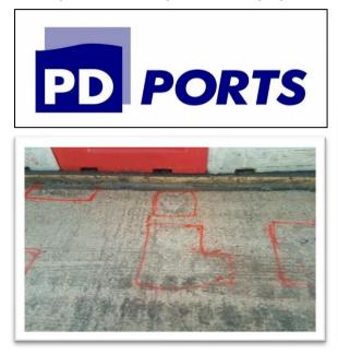
was also evident. **APA Concrete Repairs Ltd** were appointed to undertake concrete repair works to the top surface of the railway bridge deck, without disrupting crucial HGV access to and from the bustling port.
