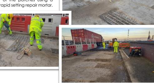
**The outcome:** The repair works to the carriageway deck of the Teesport Rail Bridge were completed on time, within budget and without disruption to the port, which was the Client's critical requirement. The use of high strength rapid deck repair materials by **APA** enabled the bridge deck waterproofing and resurfacing to commence ahead of schedule, and the
