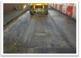
**The solution:** Working under single lane traffic management, and once the bridge deck had been exposed, the repairs were marked out and cutting and breaking out of the failing areas commenced. It was clear from the type of corrosion on the buried reinforcement that chlorides
