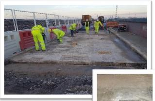
introduction of the sacrificial galvanic anodes, again by **APA**, added durability and longevity to the repaired bridge deck without adding any delay to the programme. Further solutions to the presence of chlorides were provided by **APA** but time was the limiting factor for PD Ports on this particular project.
